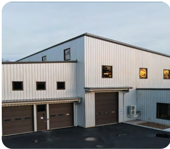
American Polyfilm Warehouse · Branford, CT
